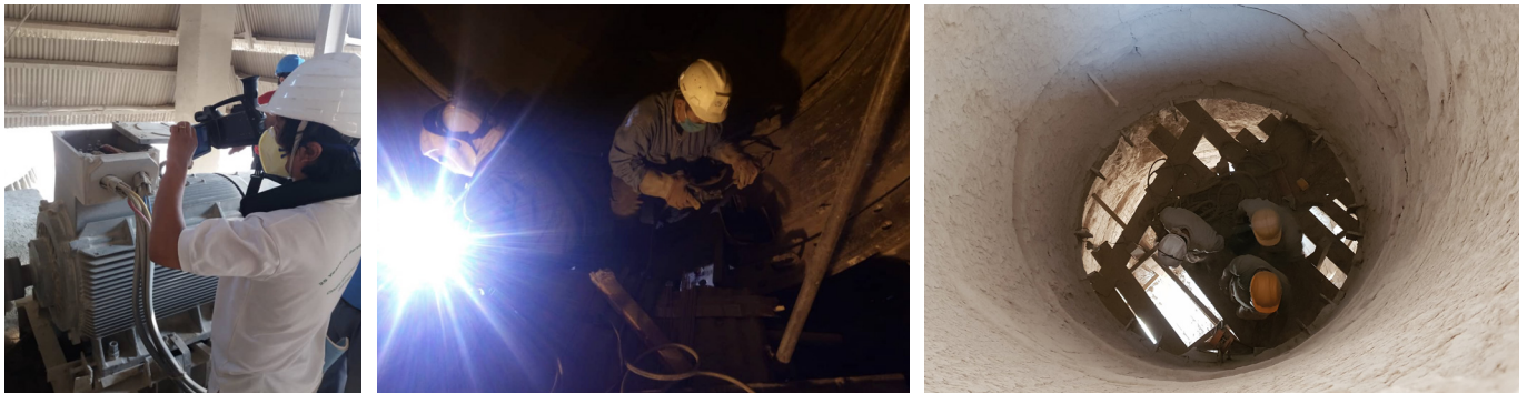
>> Introduction of condition monitoring of the plant and machineries and annual maintenance of the plant from November 14 to 29, 2018
